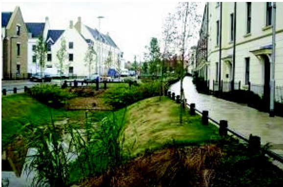
Water cycle management integrated with the built environment at Upton urban extension, Northampton.
